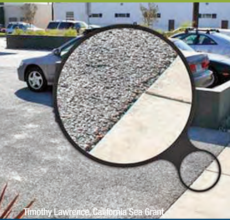
Porous concrete in Santa Monica, CA allows access and infiltration.
