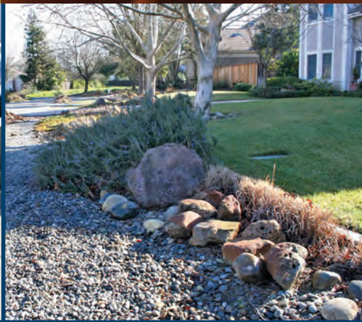
Gravel infiltration trenches within a subdivision in Davis, CA.
